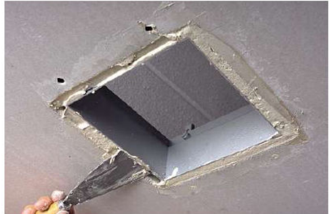
Plaster up the gap between fitting frame and ceiling.
