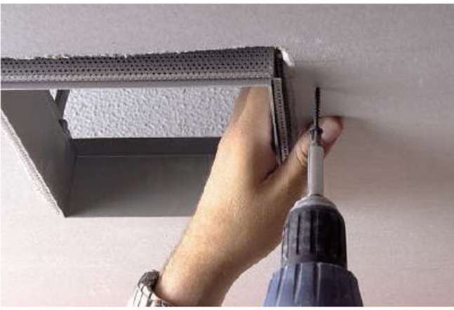
Screw the fitting frame in the ceiling cut-out with the back-mounted sieved metal sheet
