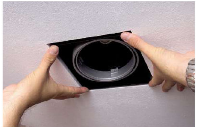
Insertion and adjustment of the bulb housing in the fitting frame with the setting screws.
